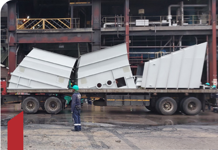
Air-Heaters Ducting & Piping Modifications
