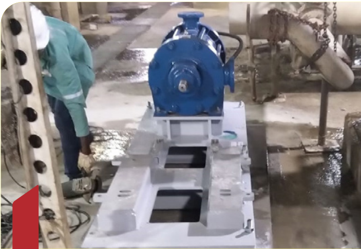
Pump Base Installation
